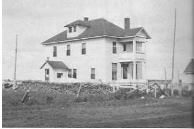
The Duclos Boys' Home or Residence, situated across the road from the first Duclos School. At the right is the little house used for some years as a residence by the Duclos School teacher H.E. Bourgoin and later occupied by the Duclos Hospital engineer John Swift.
